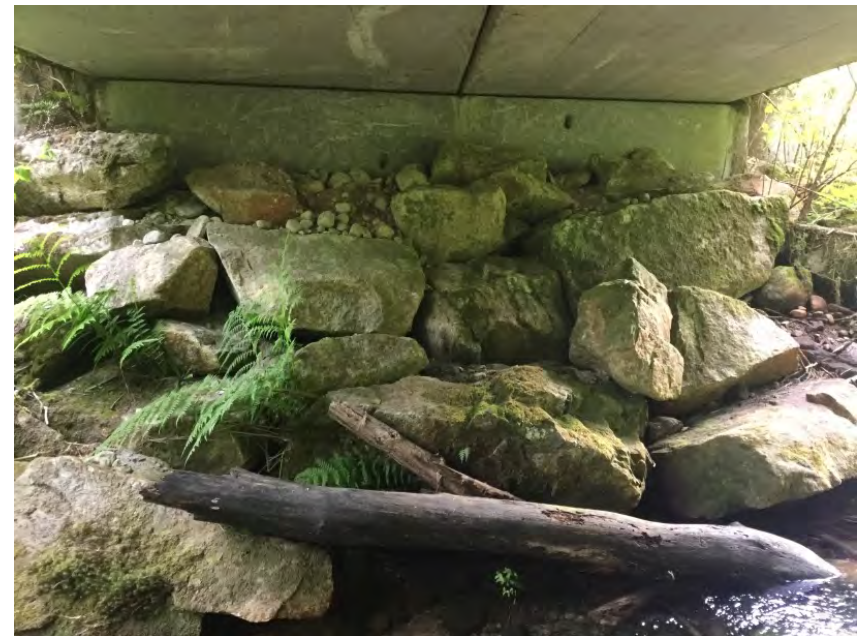
Right Bank Abutment when facing downstream
