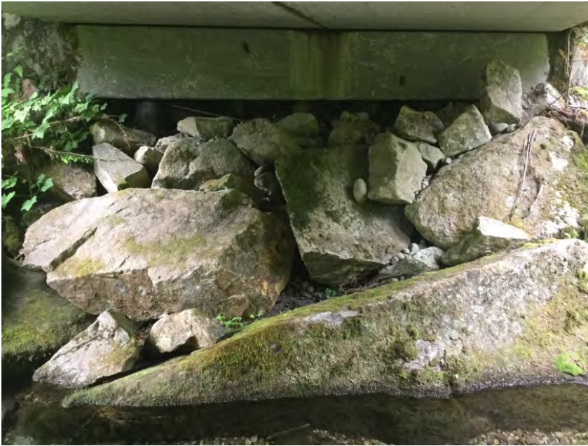
Left Bank Abutment when facing downstream
